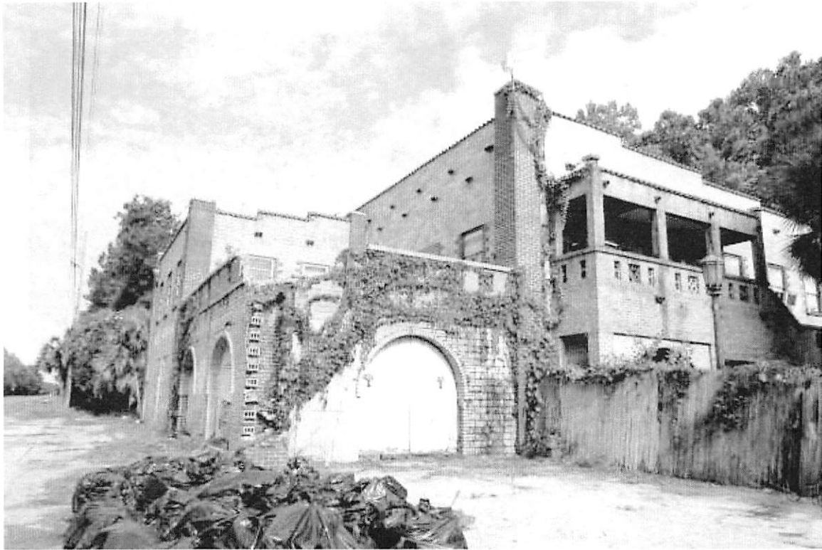
View of existing structure
